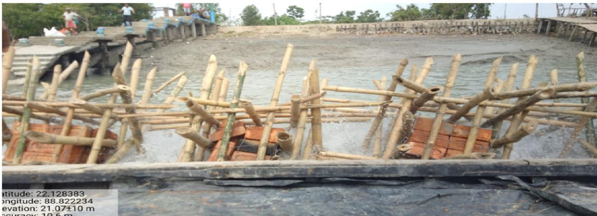
Figure 8: Porcupine structure made with bamboo after installation at STR in March, 2024
