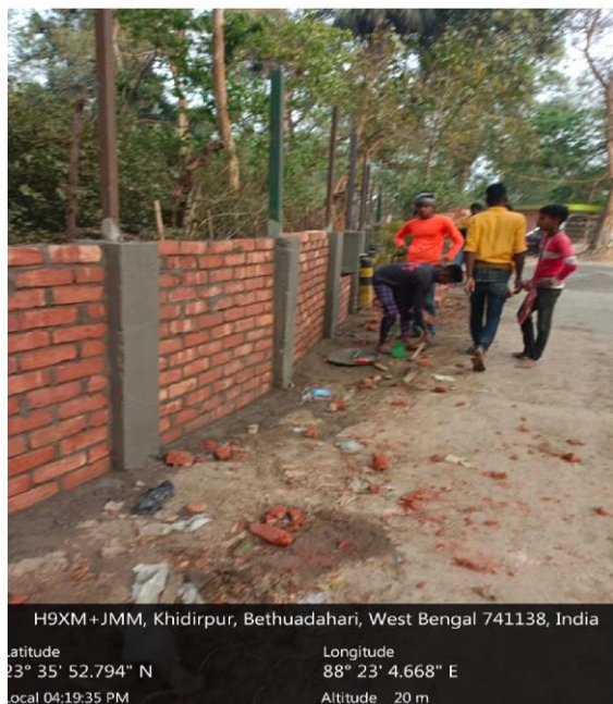
Figure 9: Brick work during development of Boundary wall and fencing at Bethuadahari Wildlife Sanctuary
