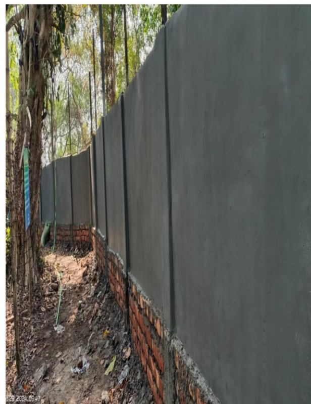
Figure 10: Boundary wall after plastering at Bethuadahari Wildlife Sanctuary
