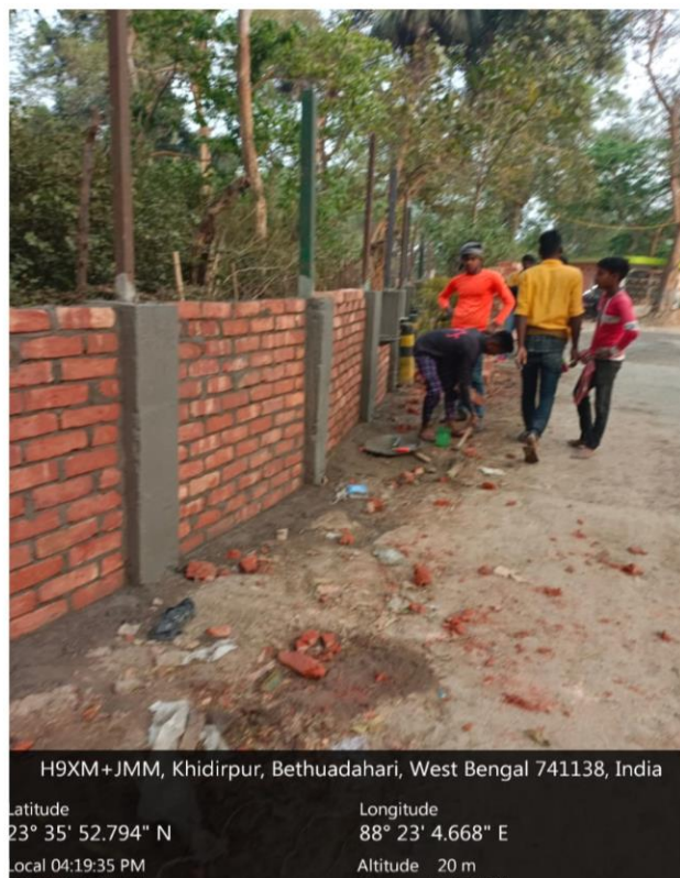
Figure 9: Brick work during development of Boundary wall and fencing at Bethuadahari Wildlife Sanctuary
