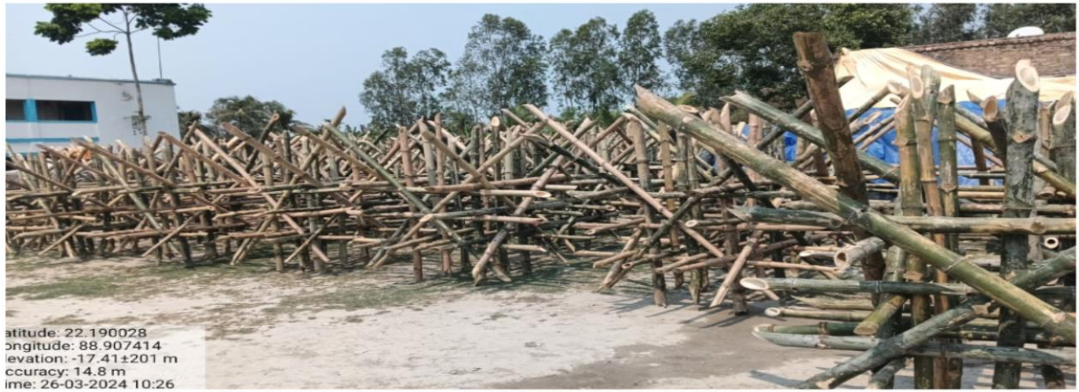
Figure 7: Porcupine structure made with bamboo before installation at STR in March, 2024
