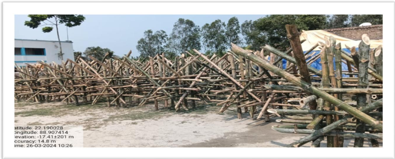
Figure 7: Porcupine structure made with bamboo before installation at STR in March, 2024
