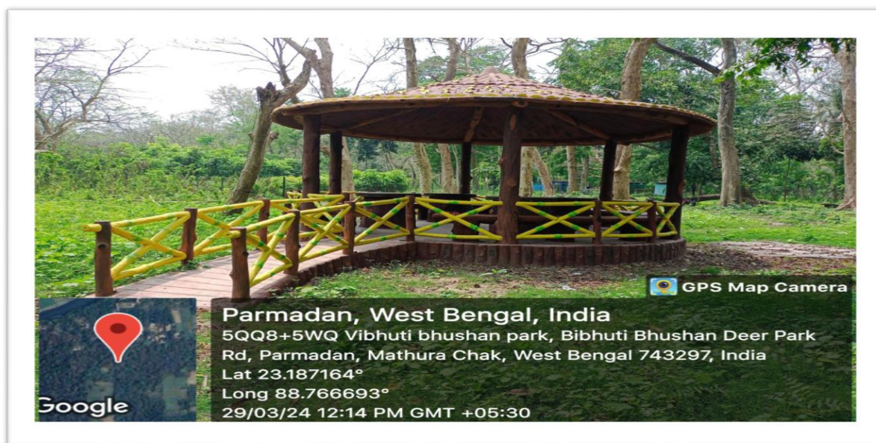
Figure 13: Construction of RCC Visitors Rest shed was done at Bibhutibhusan Wildlife Sanctuary
