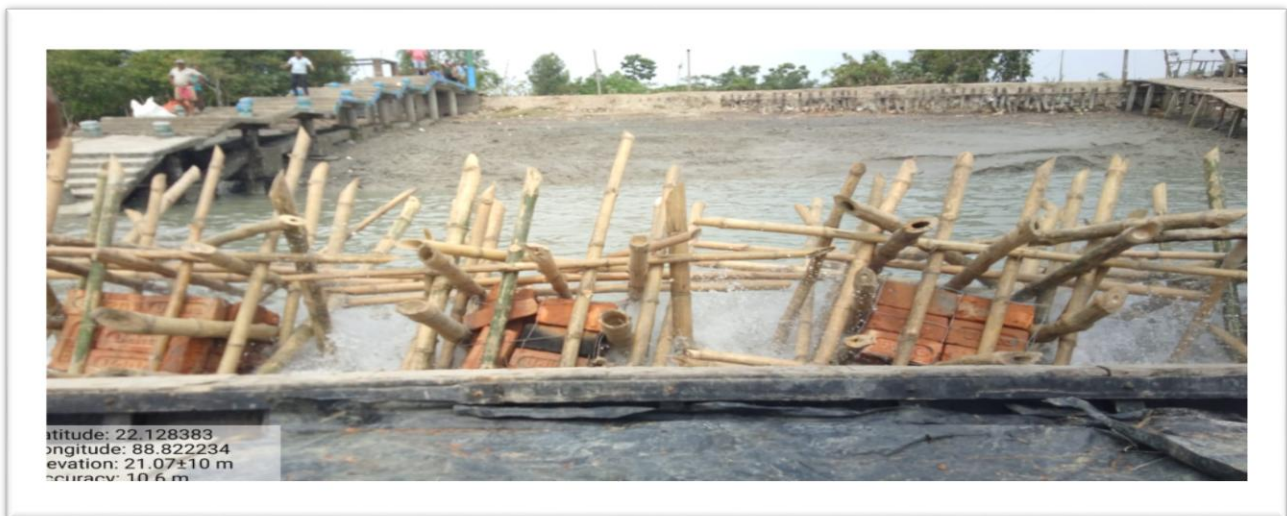
Figure 8: Porcupine structure made with bamboo after installation at STR in March, 2024
