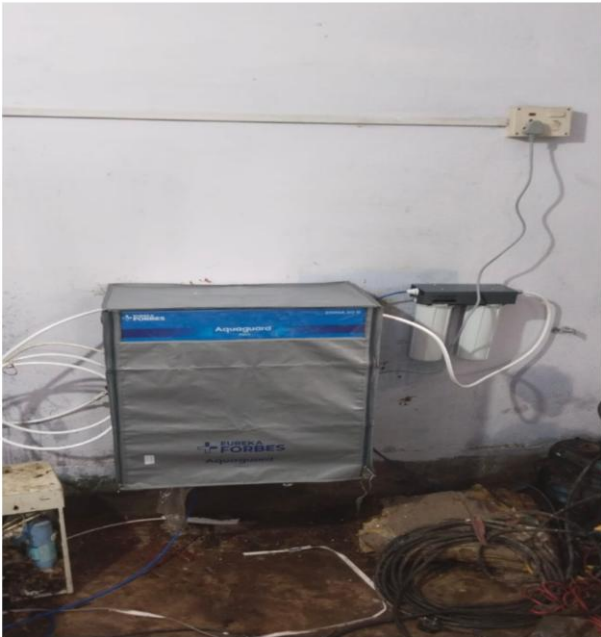
Figure 14: Installation of Submersible Pump was done at Chintamani Kar Bird Sanctuary
