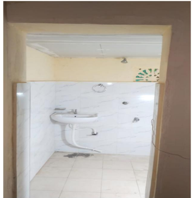
Figure 15: Construction of Staff Toilet was done at Chintamani Kar Bird Sanctuary
