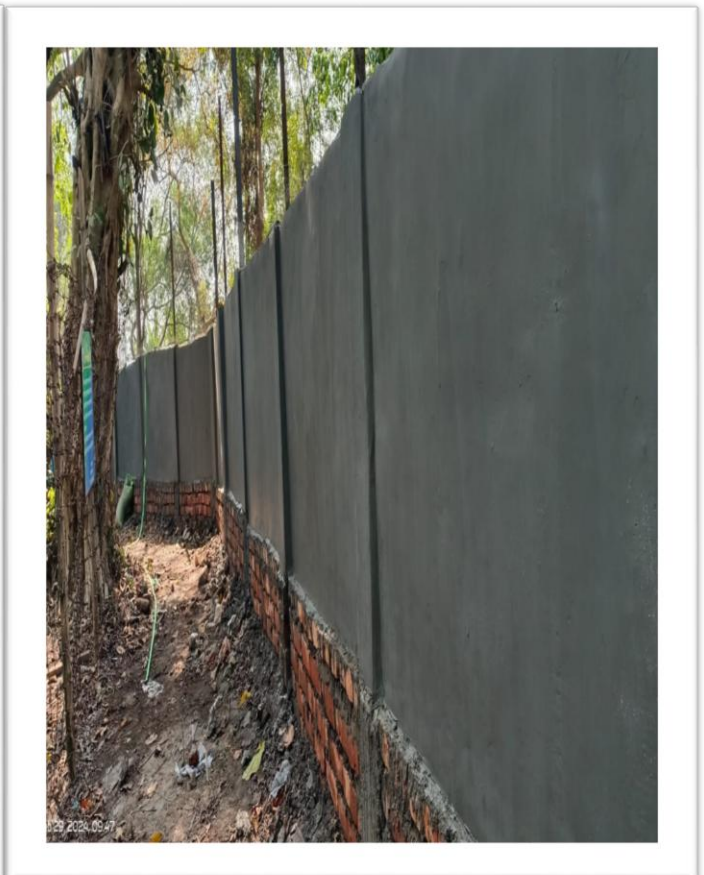
Figure 10: Boundary wall after plastering at Bethuadahari Wildlife Sanctuary
